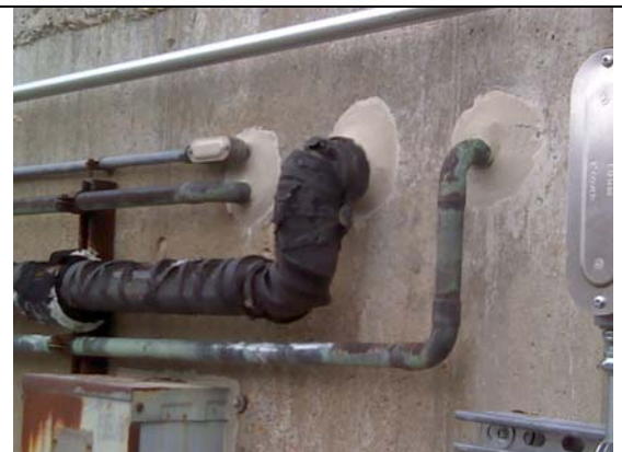
"B" Sealant installed around penetration
