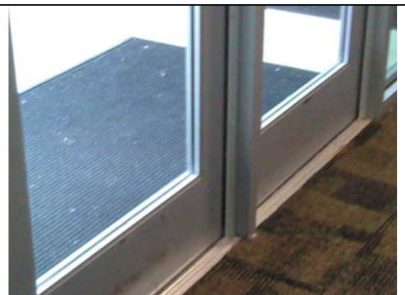
“HS 2-3” Door seals installed
