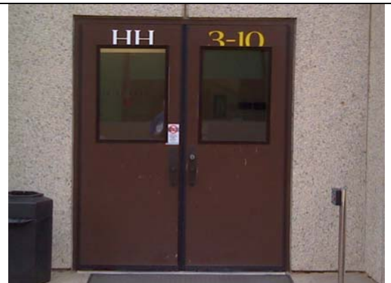
"HH 3-10" Door seals installed
