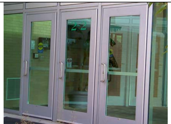
“HS 2-2” Door seals installed
