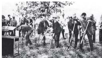
Ground Breaking - September 3, 1969
