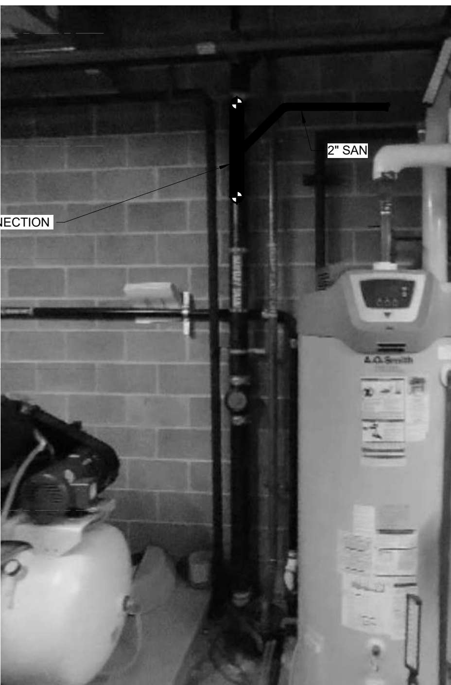
2 BASEMENT - SANITARY RISER - PLUMBING NO SCALE
